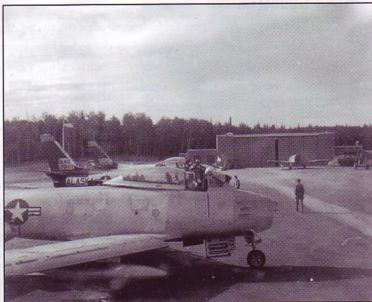
F-86 ON THE FLIGHT LINE IN FRONT OF THE ORIGINAL FIGHTER HANGAR
